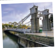
Figure 13.23 The Cavenagh Bridge over the Singapore River
